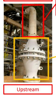
Corrosion from this pipework section deposited at downstream of flame arrestor (FA)
